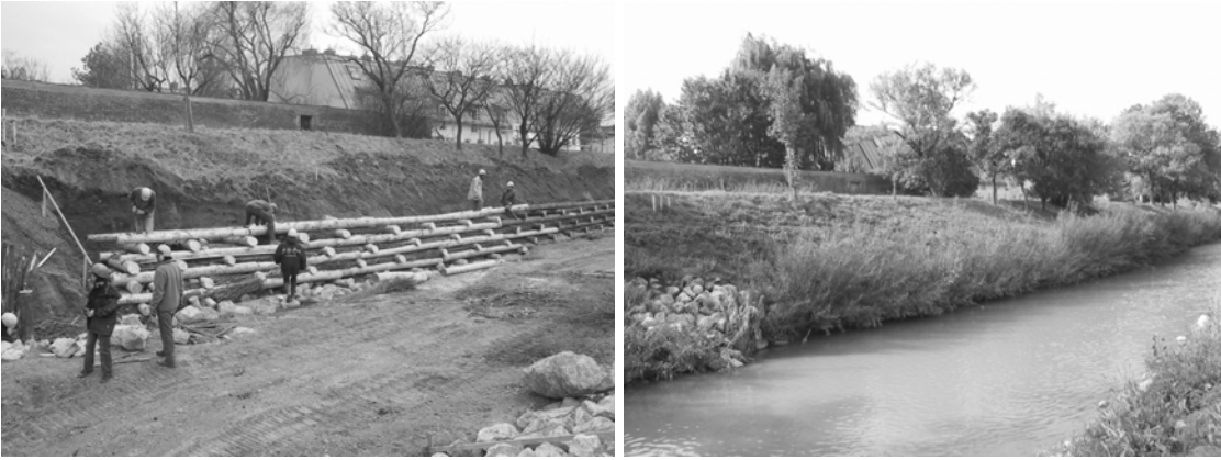
FIGURE5: Construction of vegetated crib wall (left) and 2 years after (right)
