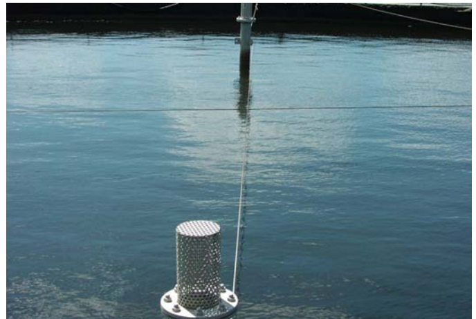
Figure 7: SBR – Settle Phase
