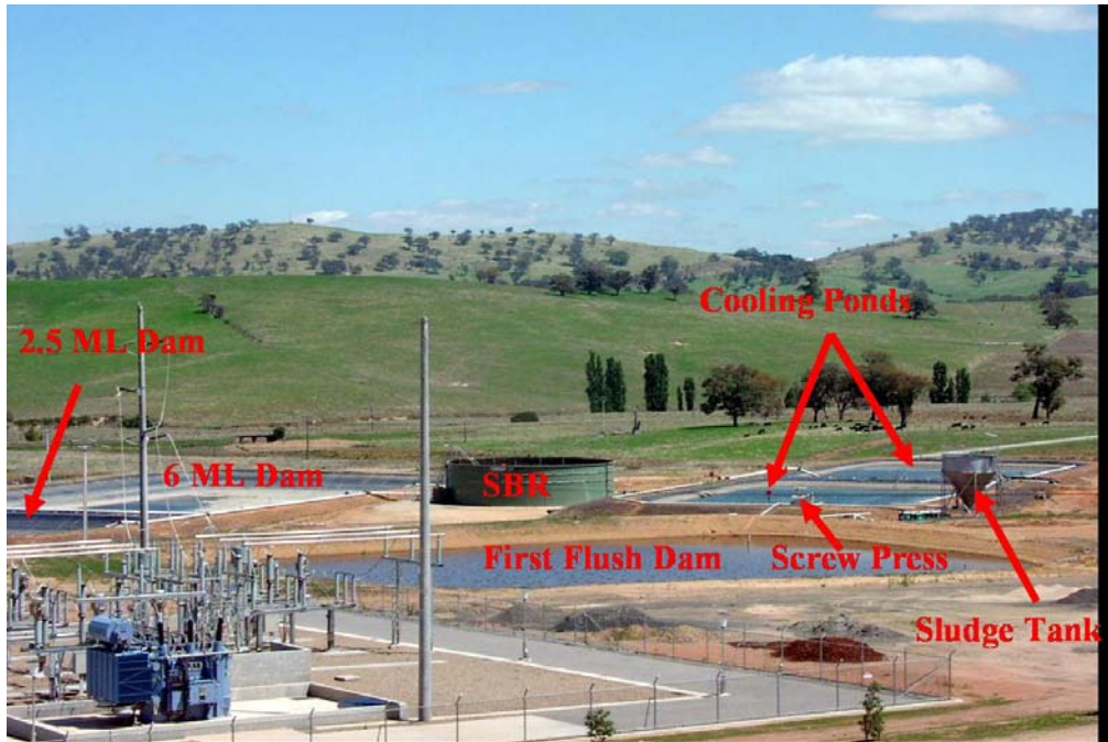
Figure 5: Waste Water Treatment Plant
